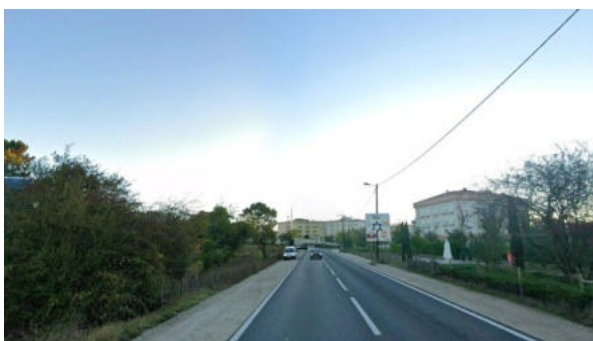
Avenida João XXIII
